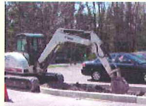
1. (above) Site is excavated.
