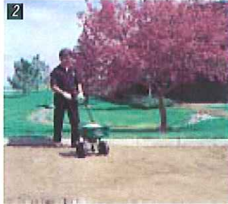
2 Apply Hydrogrow mixture.
