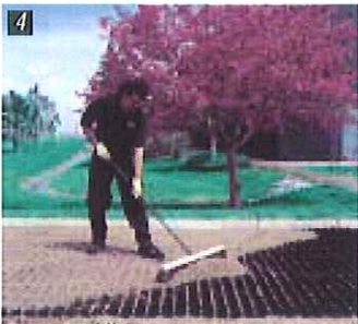
4 Fill rings with clean sharp concrete sand.
