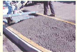
4. (above) Concrete is leveled with a screed.
