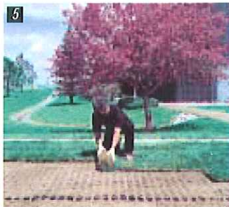
5 Hydroseed or lay sod.
