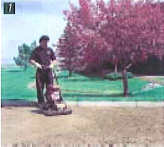
1 Place and compact sand and gravel base course.
