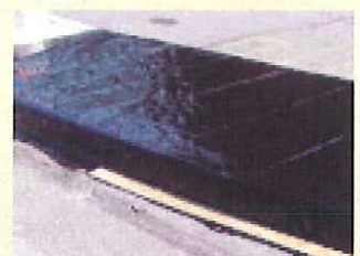
4. (above) Concrete is leveled with a screed.
