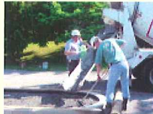
3. (above) Concrete is poured and spread.
